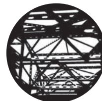
SR-6054 On A Bridge
